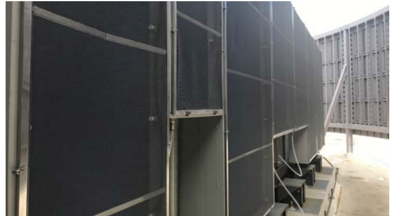
INNOVATIVE MECHANICAL UPGRADE PROJECT EVAPORCOOL INSTALLED ON OUR LONG BEACH CAMPUS
