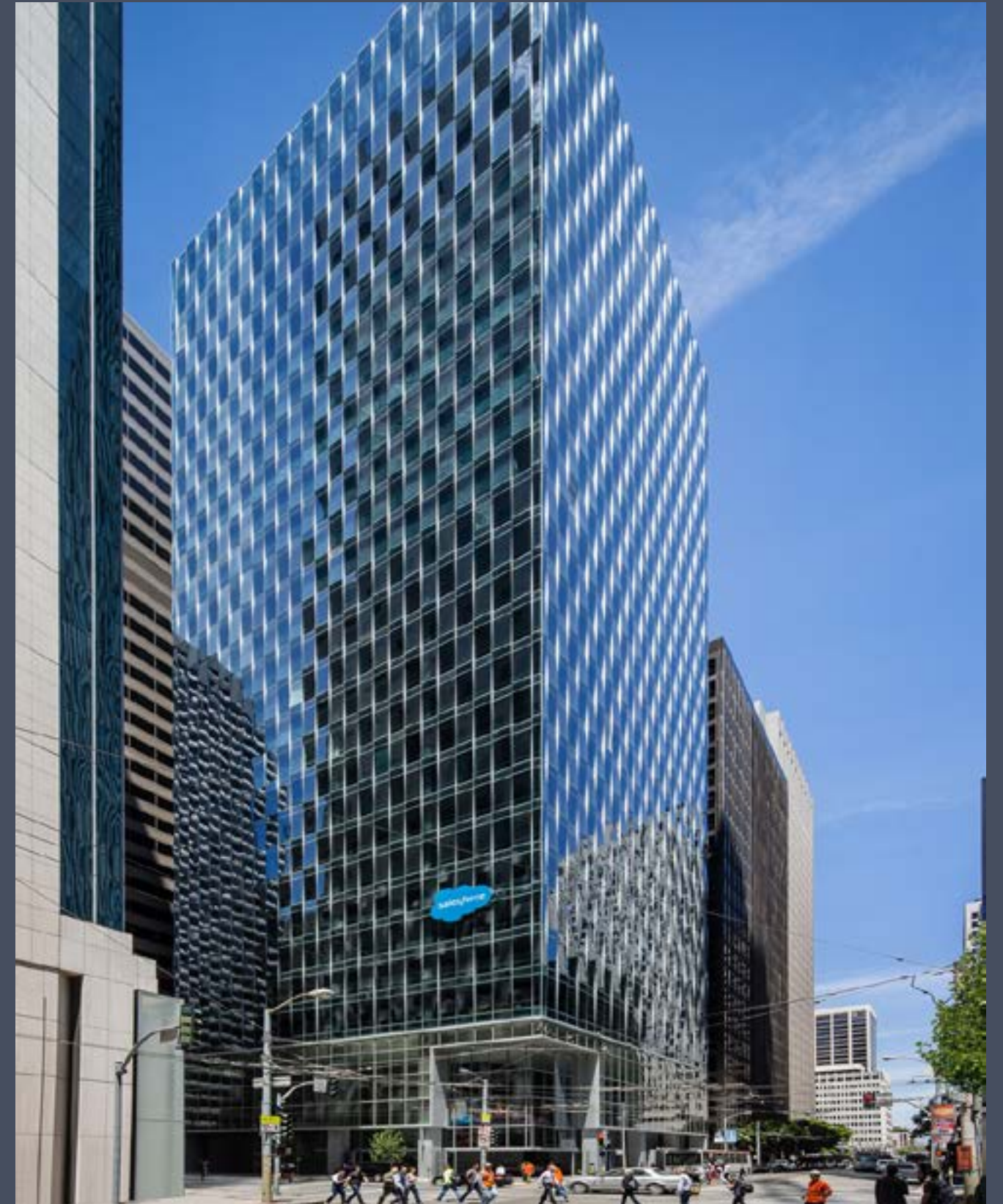
350 MISSION STREET – SAN FRANCISCO, CA // LEED PLATINUM, ENERGY STAR, FITWEL, TRUE ZERO WASTE
