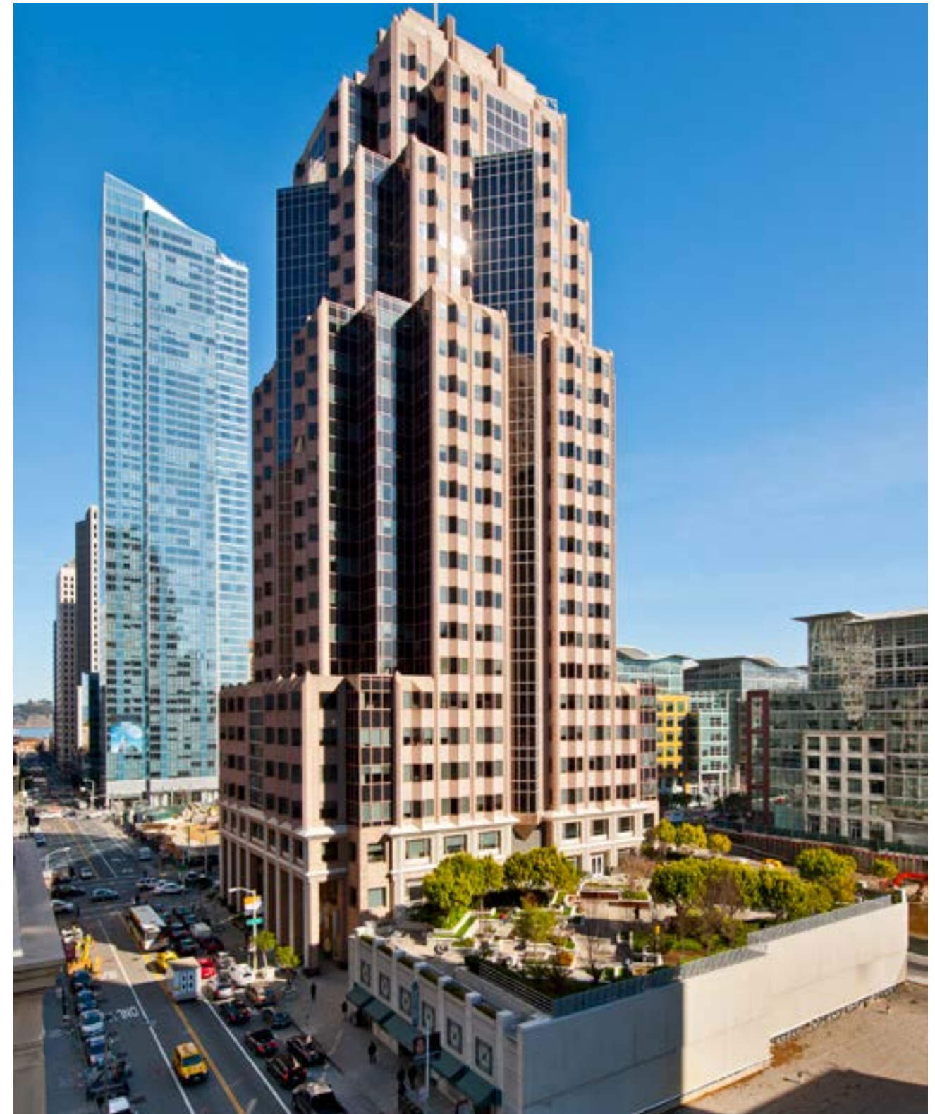
100 FIRST ST – SOMA, SAN FRANCISCO, CA // LEED GOLD, ENERGY STAR, FITWEL
